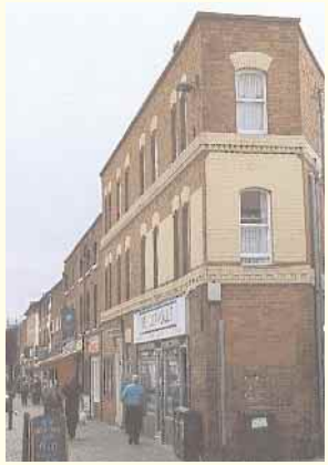
The 'flat iron' building at the head of Swan Passage in the early 21 st century.
