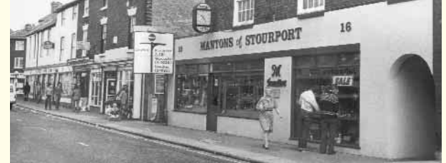
Mantons jewellers in 1974 after the integration of numbers 15 and 16. Note the arch entrance extreme right. (see below)
