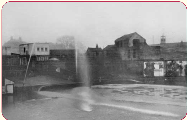
Engine House, right of centre of photograph. Picture taken from what is now the Riverside Amusements Car Park.
